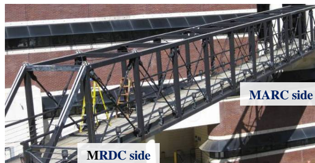
Figure 1. Picture of the space frame bridge on Georgia Tech campus.
