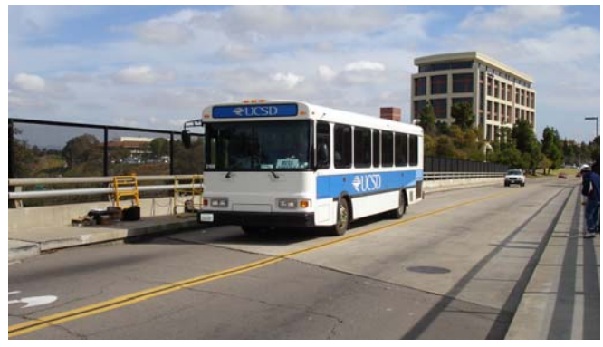
Figure 6. A photograph of an UCSD bus crossing the bridge. It can be seen that the Voigt Bridge only experiences low levels of traffic, where usually, only one vehicle passes the bridge at a time.
