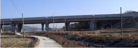
(b) Side view picture of the bridge.
