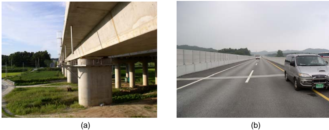
Figure 2 – Geumdang Bridge, Icheon, Korea: (a) side view; (b) top deck view
